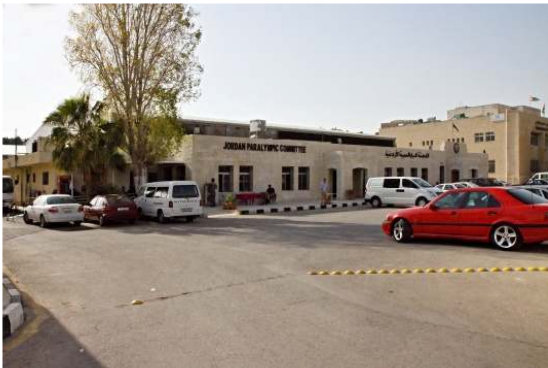
The entering part of the Prince Ra'ad Bin Zeid Complex .
